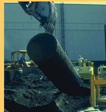
Photo 2: UST being removed
